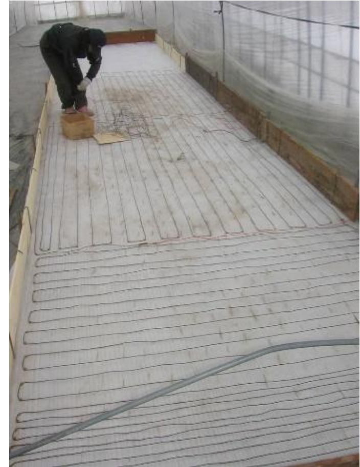
Making Electric- heated bed
