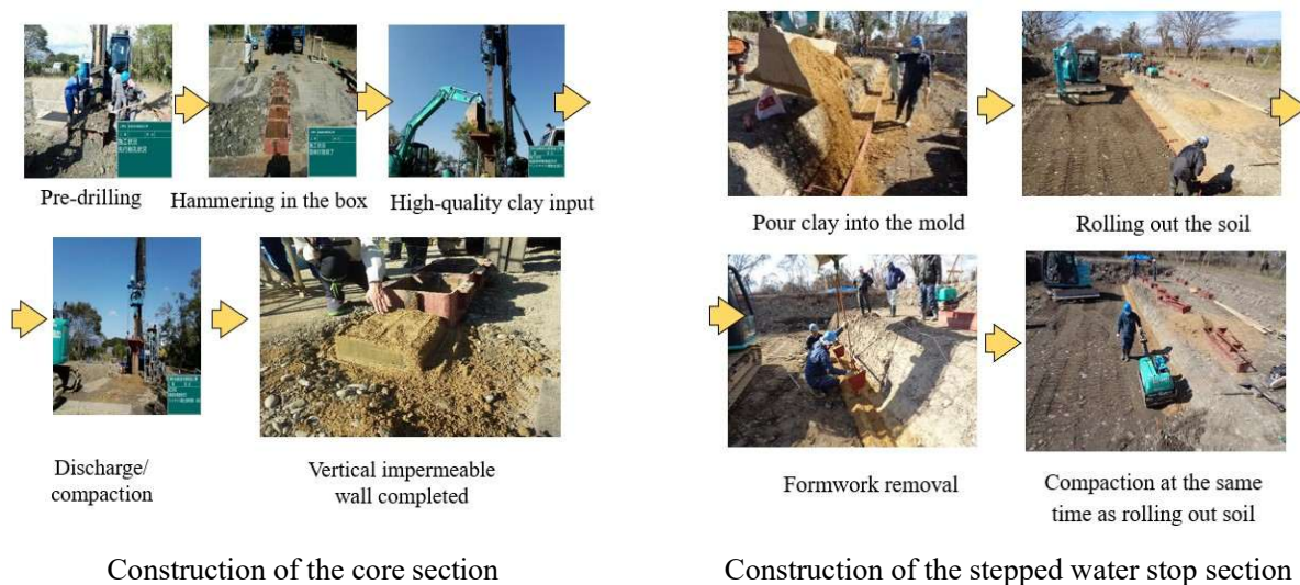
Figure C.5 Outline of bentonite mixed soil method
