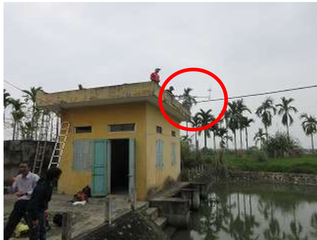
Water level sensor at An Hoa PS (An Hoa PS upstream)
