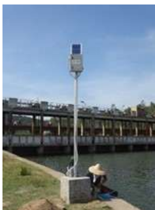
Photo 4.2 Example of installation of ICT communication equipment with anti-theft measures taken into consideration
