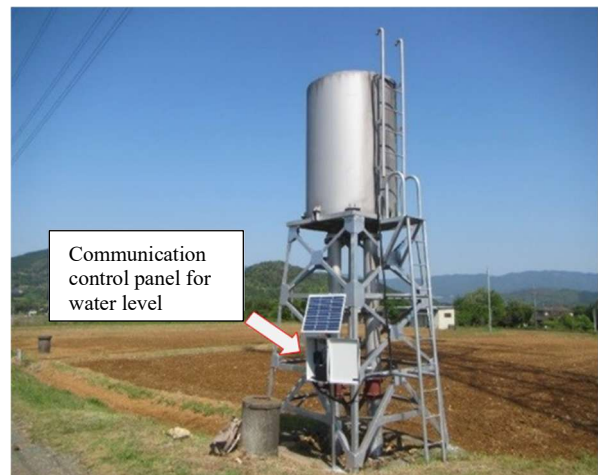
Figure 2.5 Objects of monitoring and control (left: farm pond and pumping station, right: water level monitoring of water tank) (NIRE. 2019)
