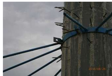
Photo 4.2 Example of installation of ICT communication equipment with anti-theft measures taken into consideration
