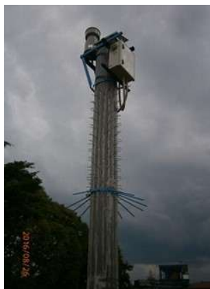
Photo 4.2 Example of installation of ICT communication equipment with anti-theft measures taken into consideration
