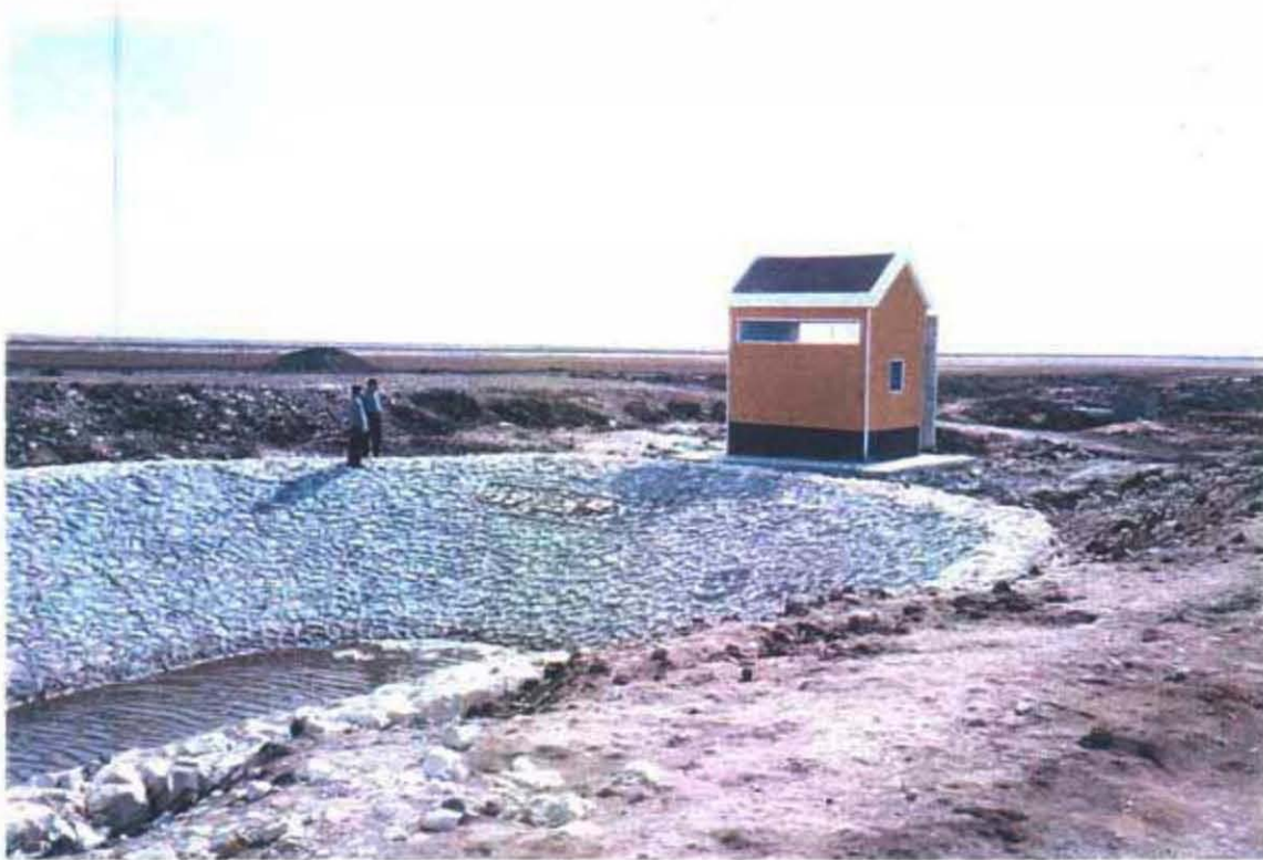
On-farm irrigation pumping Station
