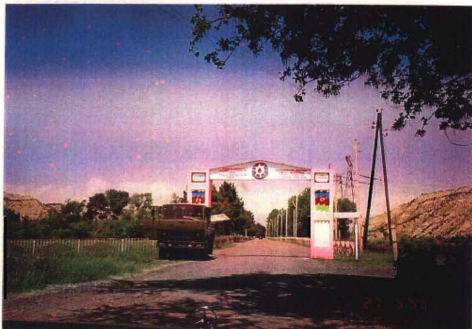
Agdash Irrigation System Office
